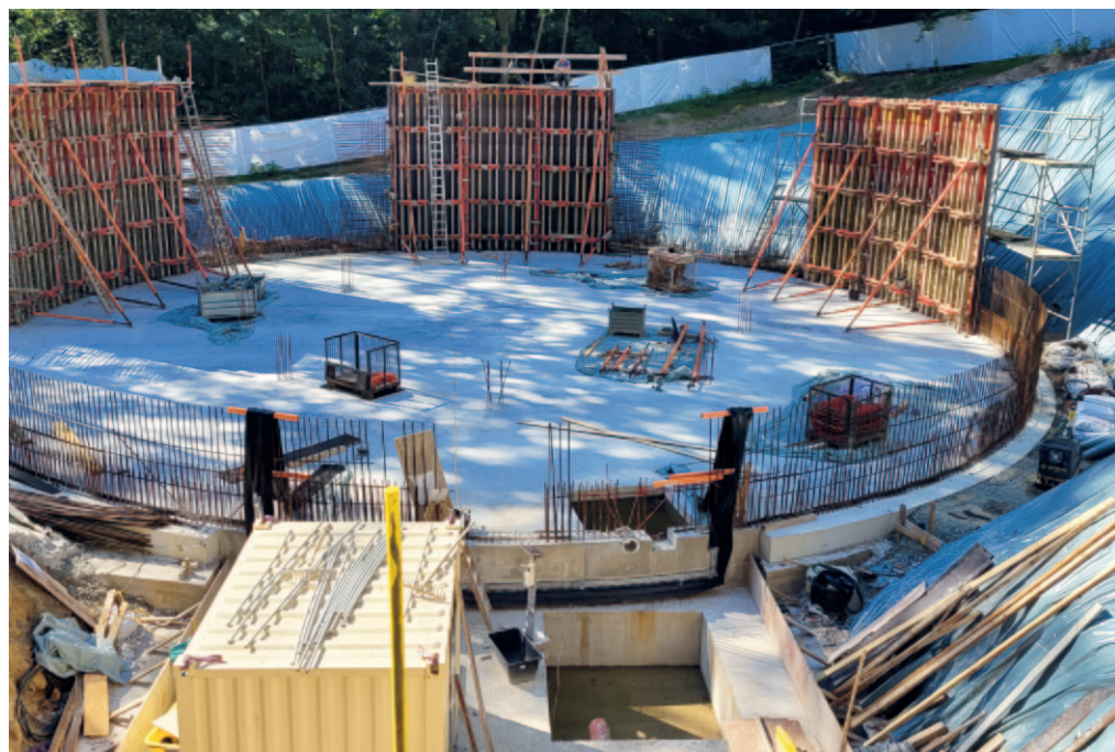
HB Kirchberg – Betonage Wandelemente
